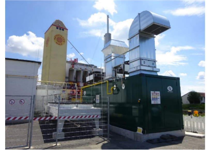
The "H 2 CHP agenitor 406 SG" from 2G Energy, based on standard CHP adapted for optional use of pure hydrogen [2G 2019]
