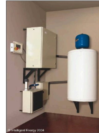
Left: Intelligent Energy 2 kW fuel cell. Initially with hot water tank, later replaced by heat exchanger
